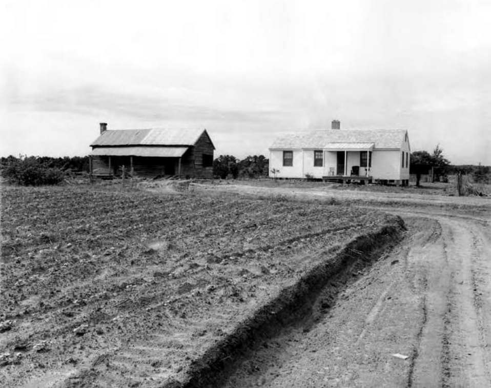
Figure 6: Old and new house at Flint River Farms
